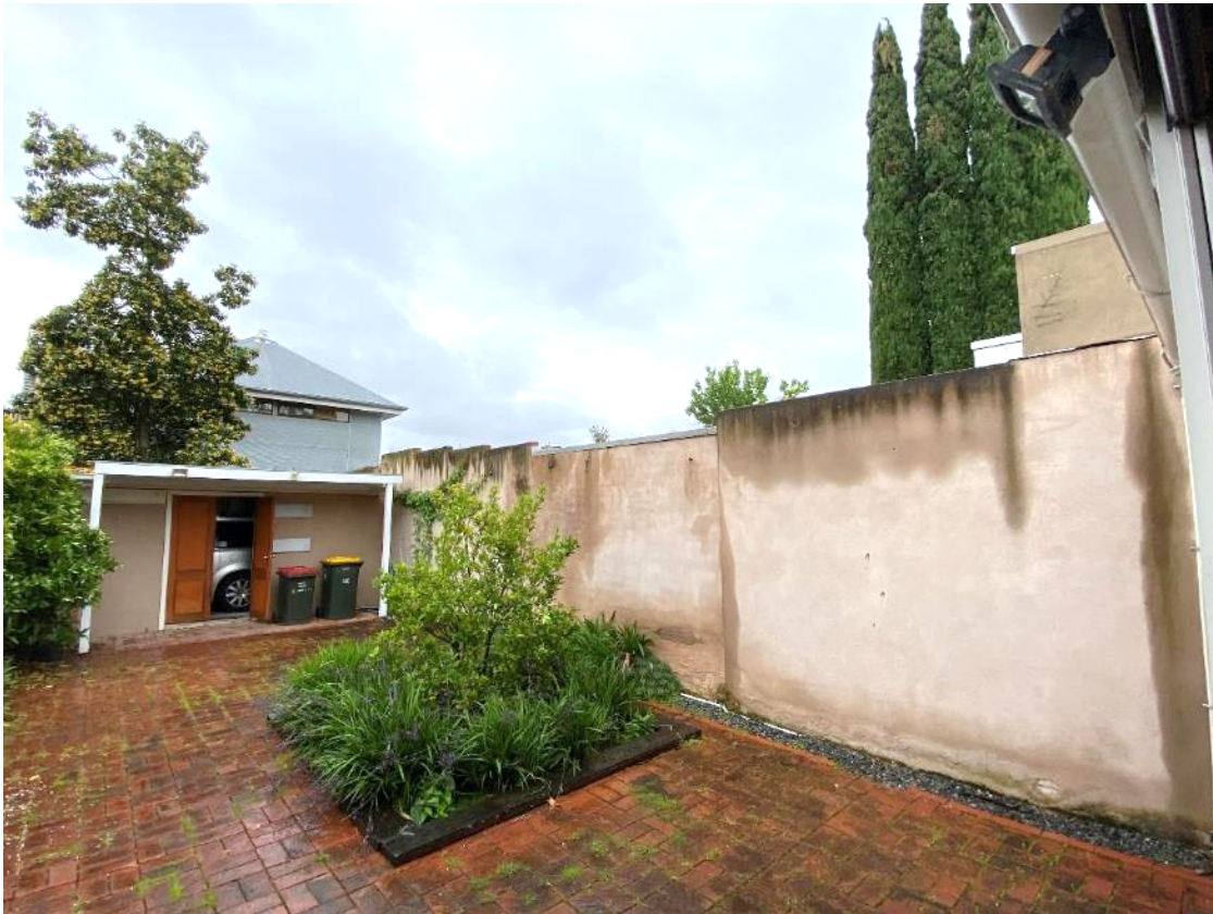
Photo 3.5 – private open space and northern boundary wall
